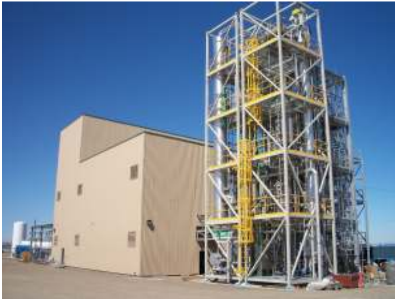
Construction of IBR facility
